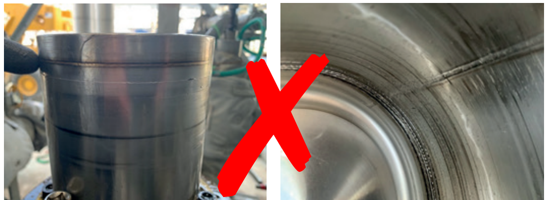
Fig. 12: Containment can Left: Groove extends over the entire wall thickness Right: several deep grooves in succession
